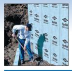
Specially designed for exterior foundation walls, STYROFOAM™ Brand PERIMATE™ Insulation has grooves that channel water down to the footing drains or weeping tiles. Offers thermal insulation, protects waterproofing membrane and assists waterproofing membrane and assists drainage of subsurface soil moisture in a single step. Suitable for use in pervious, semi-pervious and practically impervious soils. Meets CAN/ULC S701 Type 4, CCMC Class A Type 2 drainage requirements.
